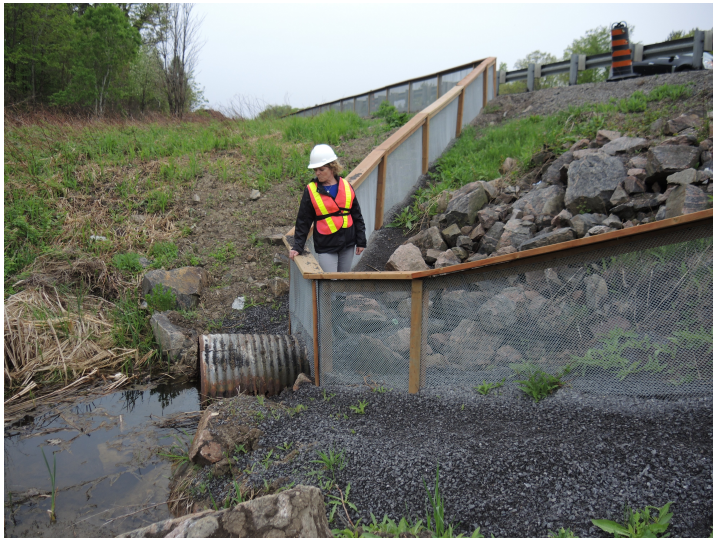
Gillian Dagg-Foster, head of the MTO's environmental section for the Ontario's eastern region, leans on fencing built to keep snakes and turtles off Highway 401.
