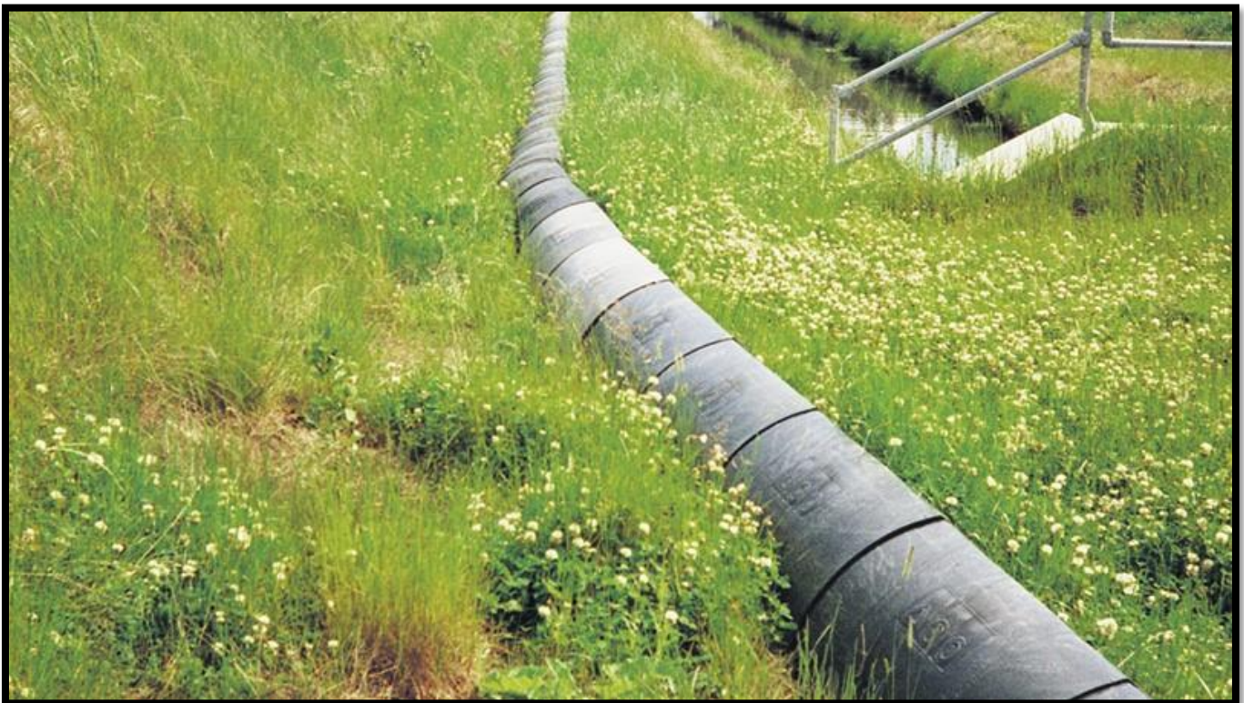
Figure 33a. ACO one-way fence panels to guide and protect wildlife. (© ACO Wildlife)
