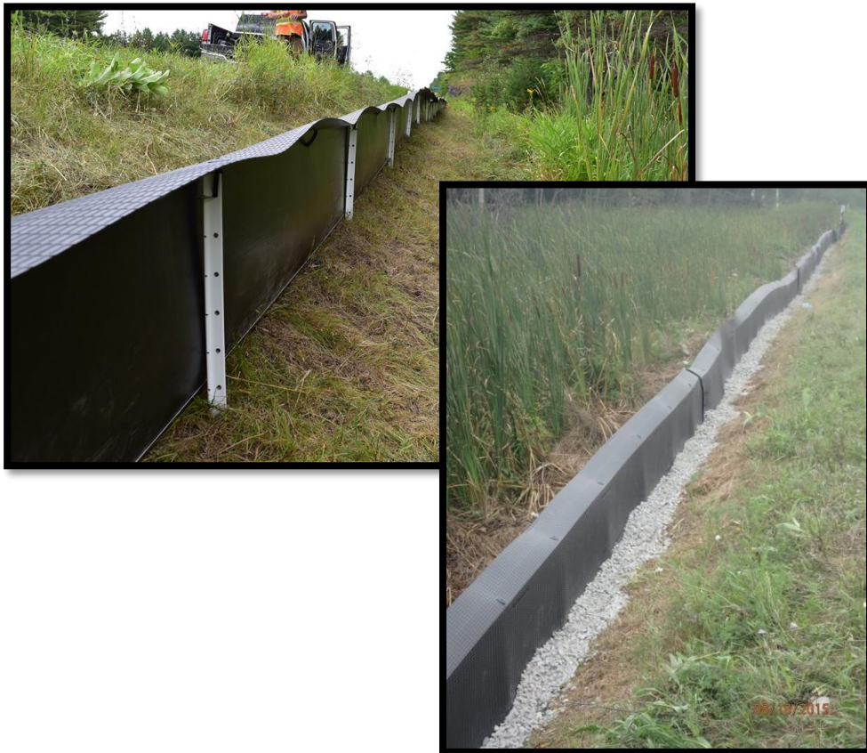
Image 1. Animex® fencing installed on Highway 7 to protect SAR Turtles. (© Eco-Kare International)
