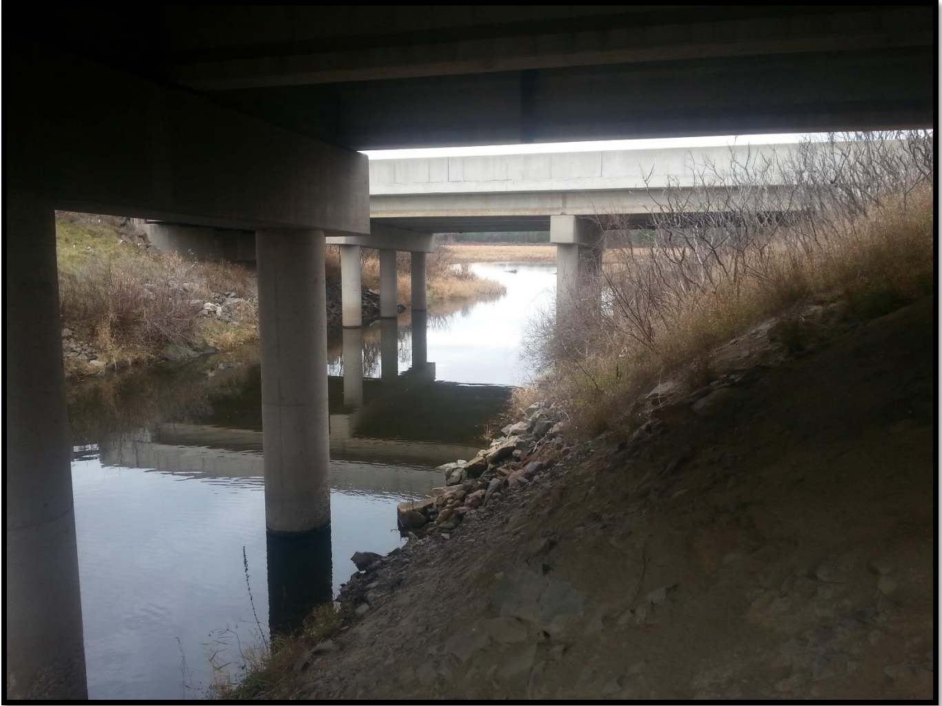
Figure 19. LaRue Creek Bridge. (© Clayton Shearer)
