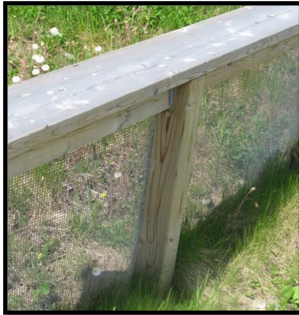
Figure 31a. Exclusion fencing targeting SAR snakes and turtles. (© Eco-Kare International)
