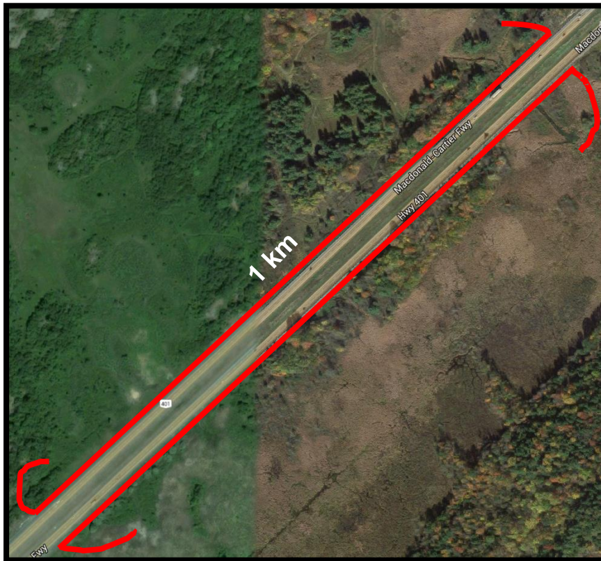
Figure 27. Recommended location for mitigation fencing (in red) for Hotspot II.
