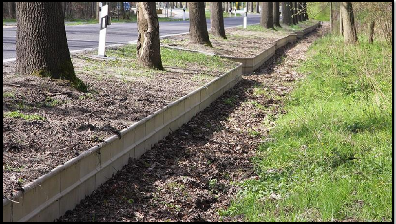
Figure 33b. ACO polymer concrete guide wall with dual protective rim to deter wildlife climbing over the top. (© ACO Wildlife)
